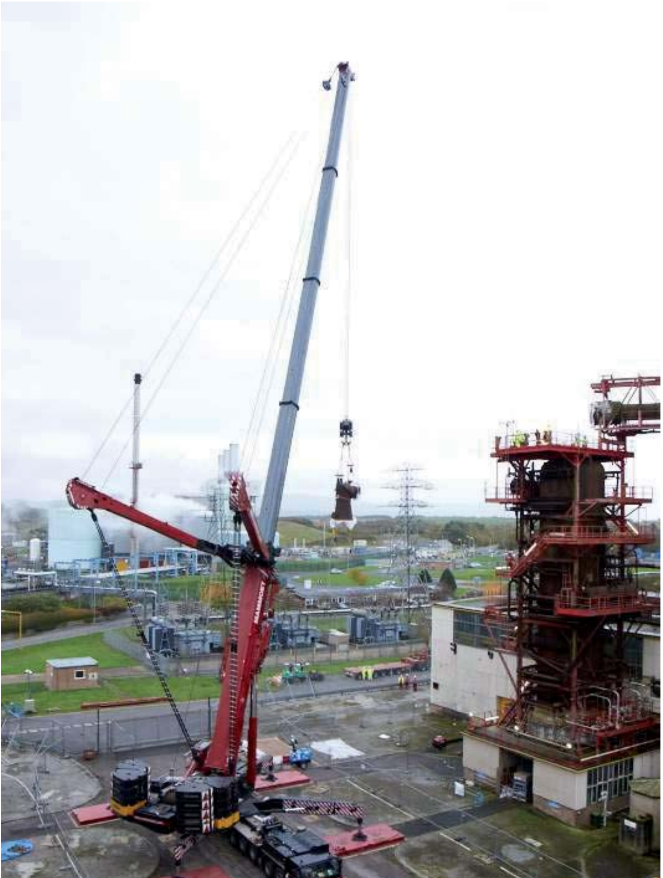
Mobile Crane lifting elbow prior to duct removal
